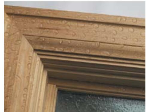
With a water-based vacuum/pressure process, virtually 100% penetration of active ingredients can protect wood from decay, water saturation, and termites. Standard dip-treated wood only protects 20–40% of the wood.
